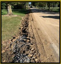
After completing the pipe, Road Crews began repairing the berm along Crossley Road. First, using soil reserves, crews filled the upper sides of the ditches using the six-way blade for the Bobcat. Once filled, the crew used the blade to compact the dirt down. Finally, the crews touched up the grading behind the skid steer using a trackhoe. This method expedited the work, allowing Road Crews to complete the entire berm along Crossley Road.
