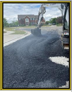
After completing the emergency repair, crews worked to finish milling in Quail Meadows subdivision before the cape seal crews arrived on 6/29.
