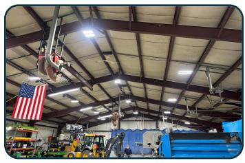
In the last week of February, crews focused on shop maintenance by replacing 11 High Bay lights. The original lights, installed in 1995, were replaced with energy efficient LED lights.
