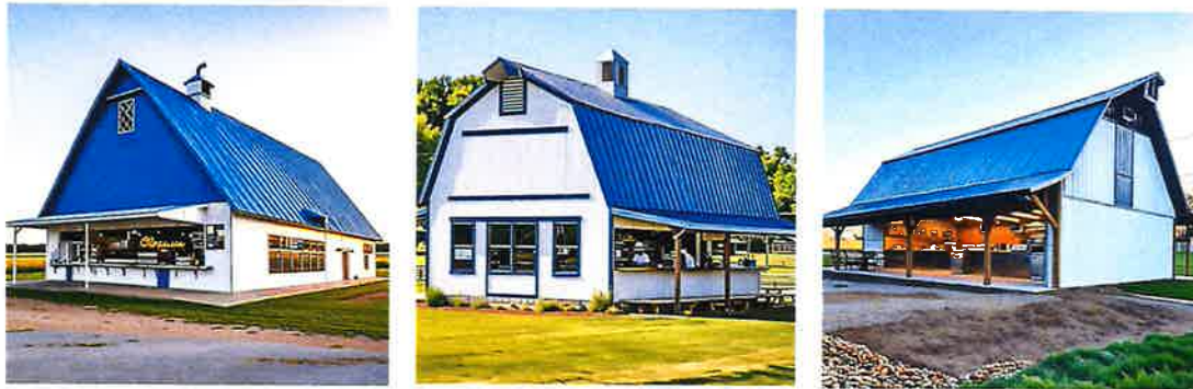
Farm Kitchen Building 40' x 80'
